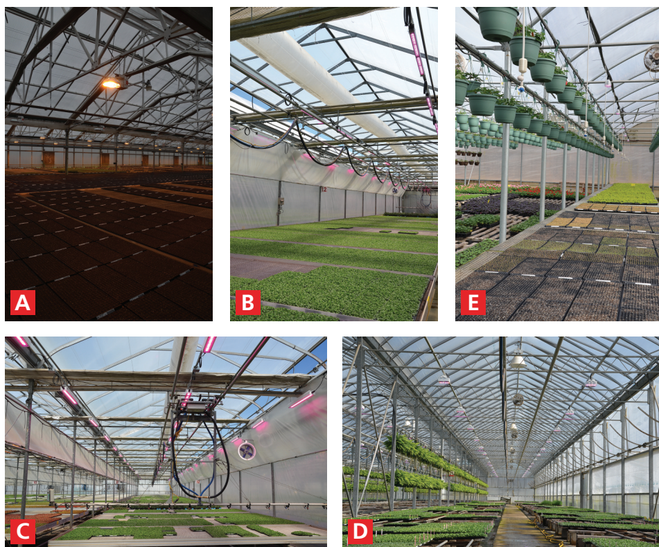
Figure 1. Supplemental lighting of young plants utilizing A) high-pressure sodium lamps, B-D) various commercially available high-intensity light emitting diode (LED) fixtures or E) LED photoperiodic lighting.
